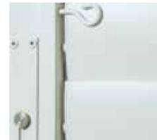
Pin used to lock louvres
